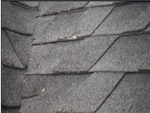
-damaged shingles
