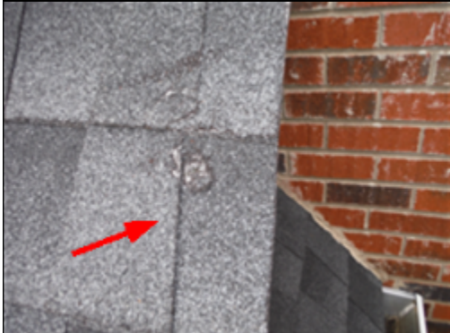
-damaged shingle
