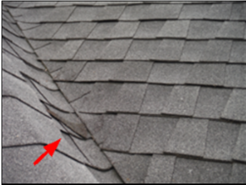
-damaged shingle
